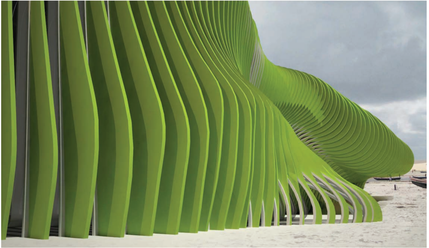
10 External view of structural frames
